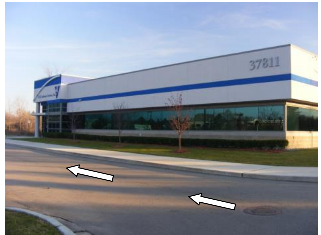
Coming from the Bank of America Directions: entrance off 12 Mile Rd
